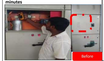
**COUNTERMEASURE:- Provided a ammeter to** monitor the current drawing by capacitor, so on
